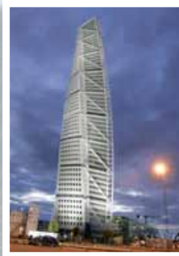
Turning Torso, a 190 m tall building for residents. Photo: Pierre Mens
